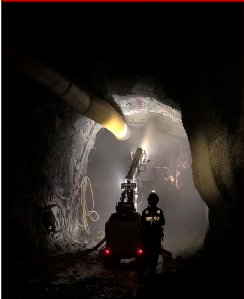
Robotic Shotcrete Machine
