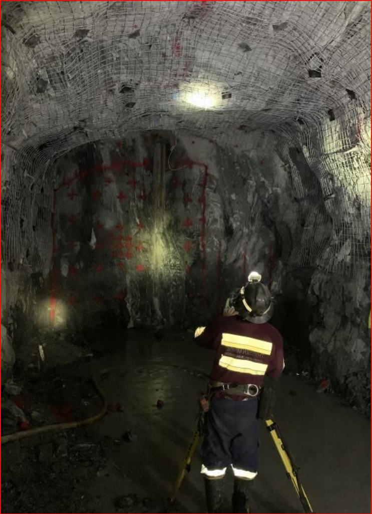
Setting out the Blast Pattern
