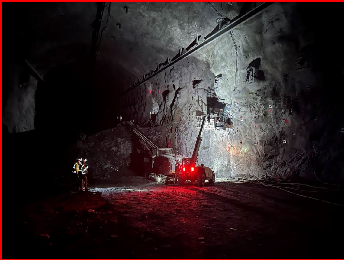
North Cavern (4850-33) CT Bolting & Grouting
