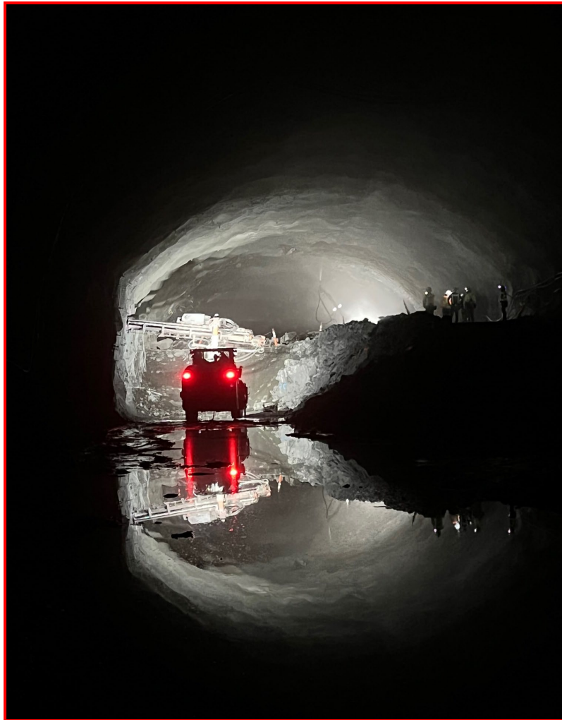
CUC (4850-36) Installing CT Bolts
