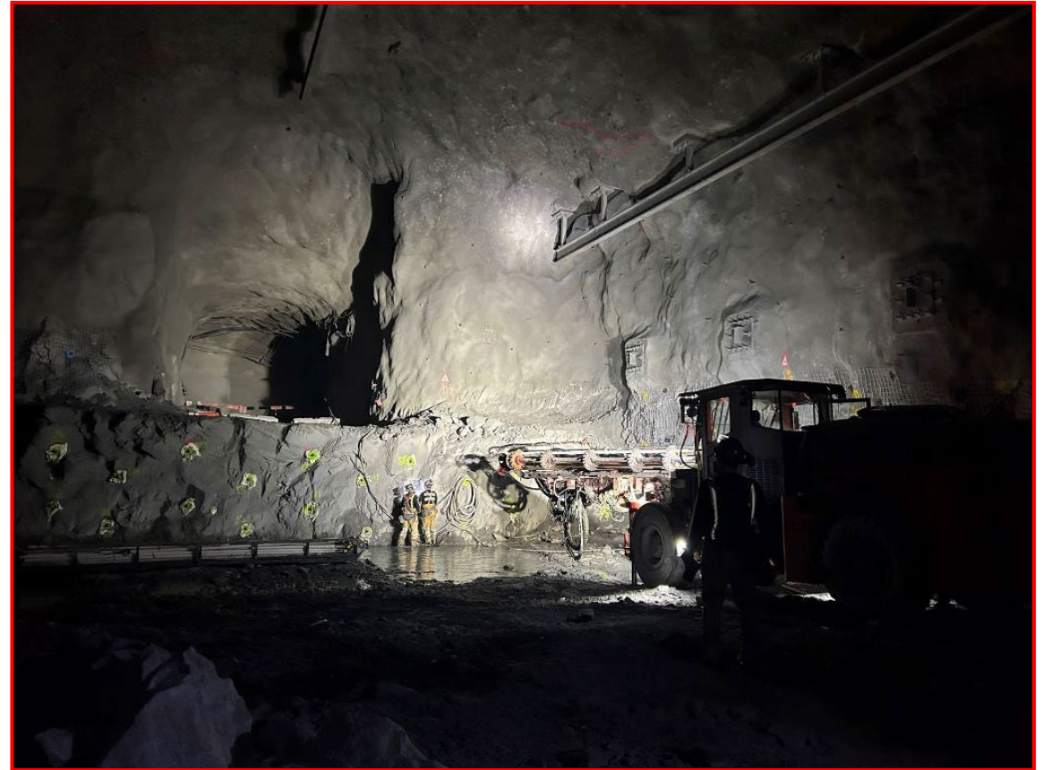
North Cavern (4850-33) CT Bolting
