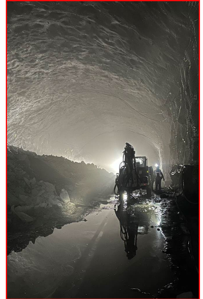
CUC (4850-36) Shotcrete Setup
