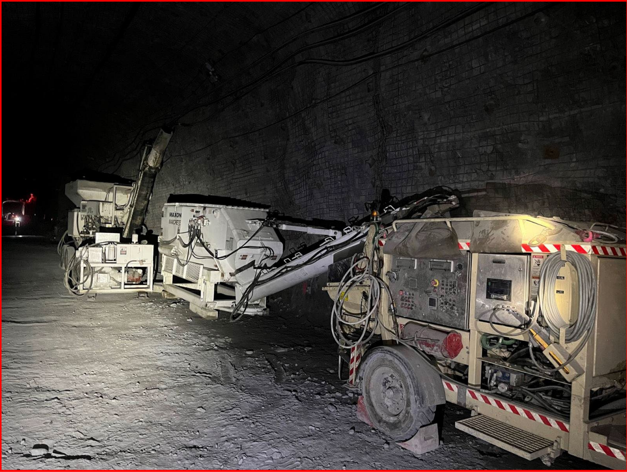
CUC (4850-36) Installing CT Bolts
