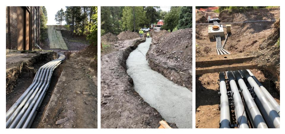
Duct Bank installed from substation to near headframe Keeping up with other work
