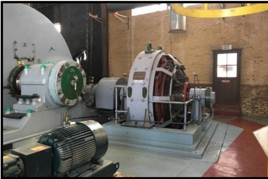
Hoist Motor Rehabilitation
