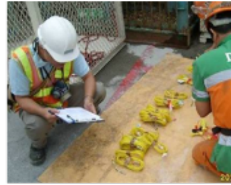
2. Remove Explosive from magazine
