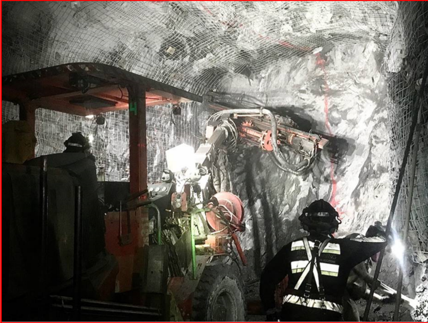
TMI Personnel Installing Ground Support (Split Sets and Welded Wire Fabric)
