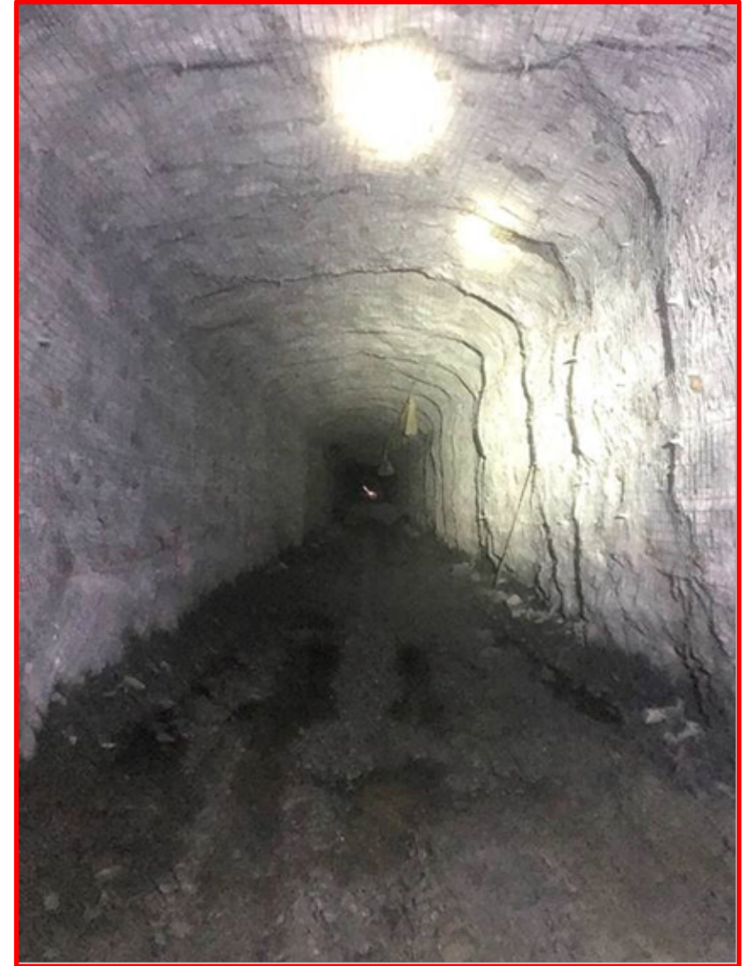
4850-02 Drift Profile Looking Towards Ross Station
