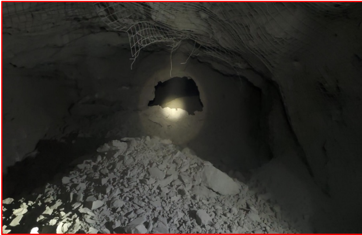
North Cavern Pilot Hole Breakthrough!!!! January 11, 2022
