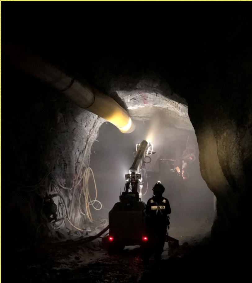
Robotic Shotcrete Machine
