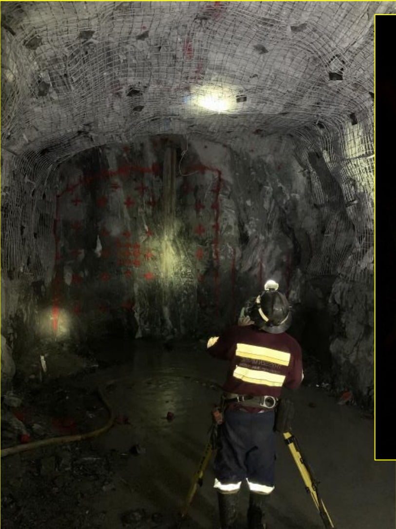
Setting out the Blast Pattern
