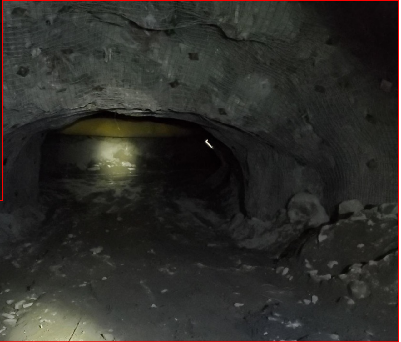
North Cavern Pilot Hold Looking East
