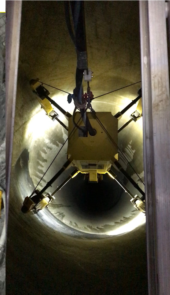
Shotcrete Robot in Raise
